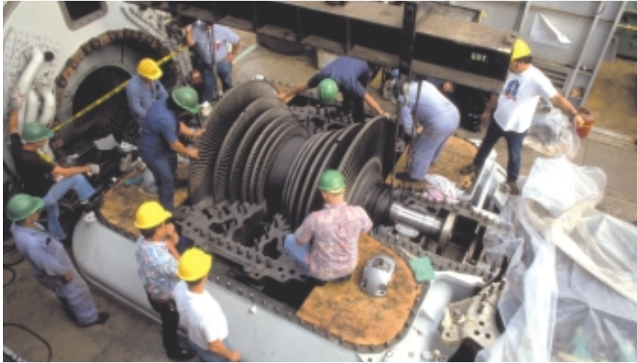
Turbine overhaul, Kahe Power Plant
